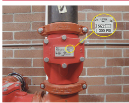
EXHIBIT 14.7 Check Valve Listed for 200 psi (13.8 bar). (Courtesy of JENSEN HUGHES, Inc.)
