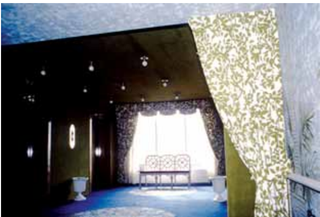
Las Vegas Hilton elevator lobby with carpetlike textile wall and ceiling finish material.
