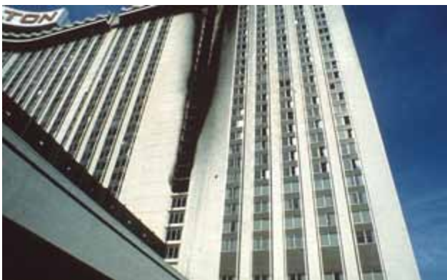
Resulting fire spread involving elevator lobbies on eighth through twenty-fourth floors.
