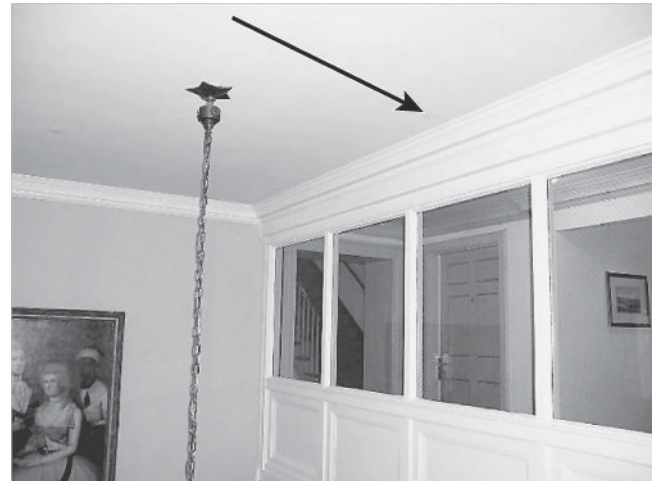
FIGURE F.3(a) Sprinklers to Maintain Glass Cooling.
