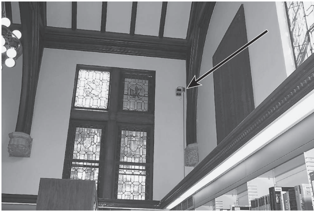
FIGURE F.4(c) Linear Beam Smoke Detector.
