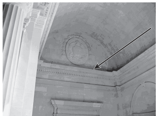
FIGURE F.3(c) Exposed Sprinkler Pipe.
