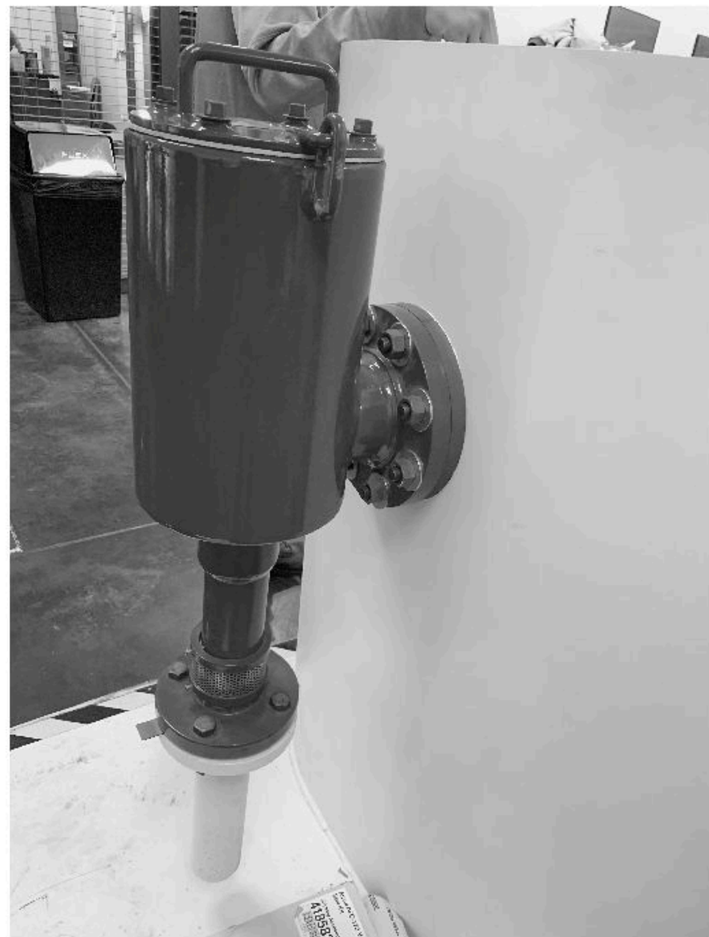
Δ FIGURE A.5.2.5.2.1(a) Foam Chamber.
