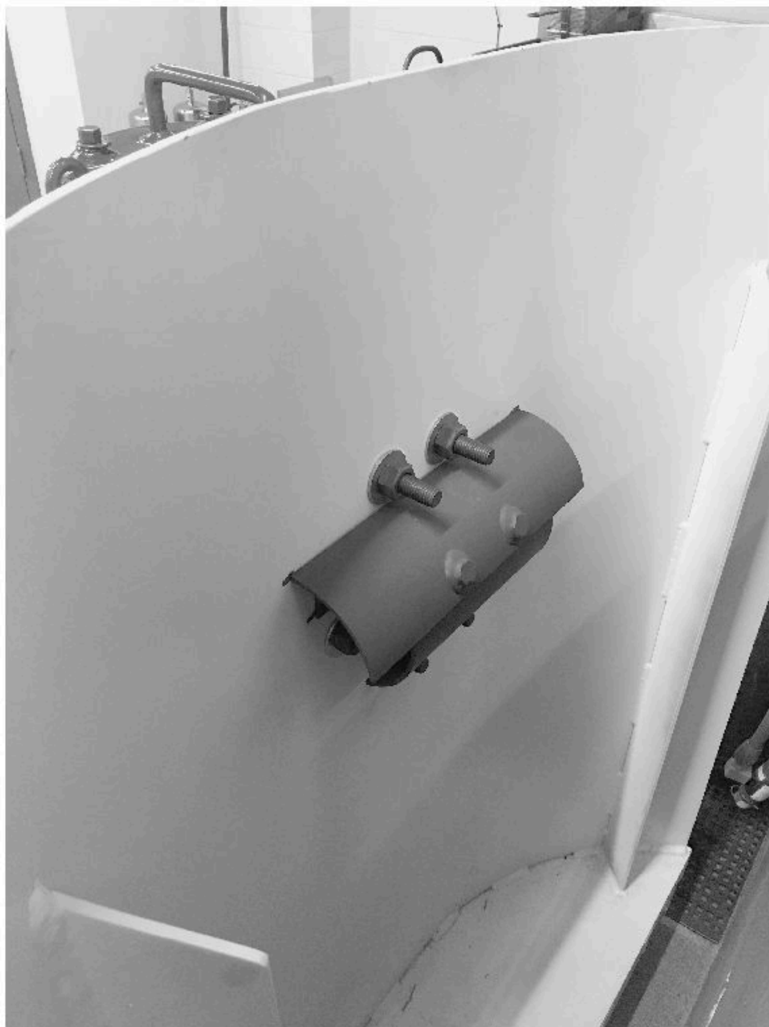
Δ FIGURE A.5.2.5.2.1(b) Foam Chamber Deflector.
