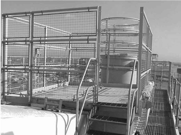
FIGURE 6-6. Top access hatch, top bag removal design
